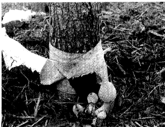
Figure 5. A potentially lethal combination at the base of this tree; tree wrap held in place by a deep mulch layer. The bark and paper wrap were water-soaked and stained, and mushrooms growing on the mulch were evidence of the saturated condition.
