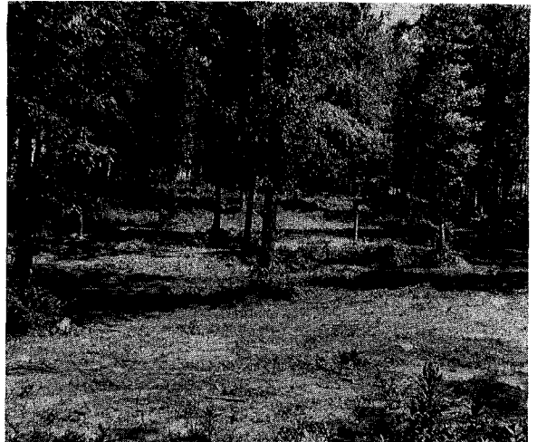
Figure 6. A stand in which the soil surface was graded by a bulldozer before houses were built. Bole wounds are noticeable, but more important, the grading severed roots and compacted the removed or added soil, thus causing damage that will result in dieback of many tree crowns within 3 years (Figure 7).
