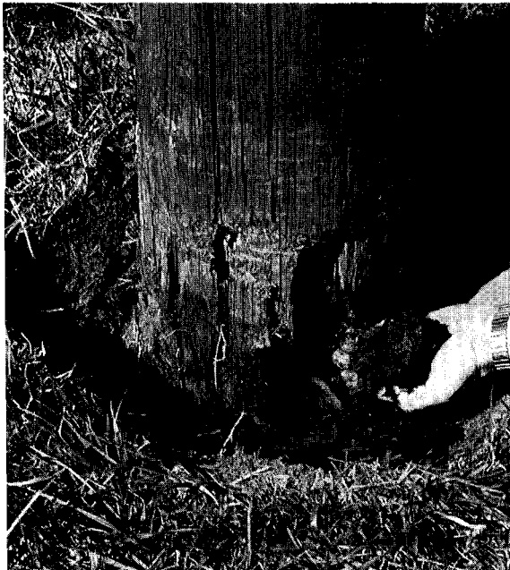
Fig. 1. External and internal decay just below groundline on a southern yellow pine pole.
