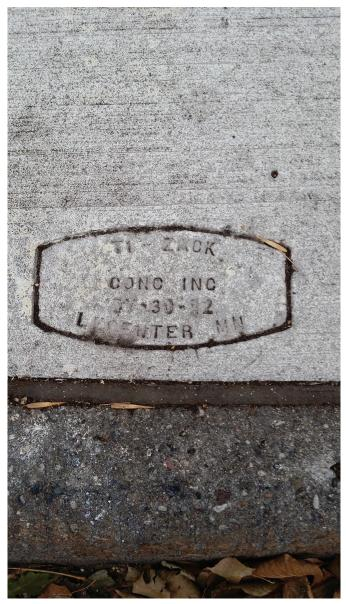
Figure 7. An example of a date stamp on sidewalk replacement/ repair. Date is 07-30-12.
