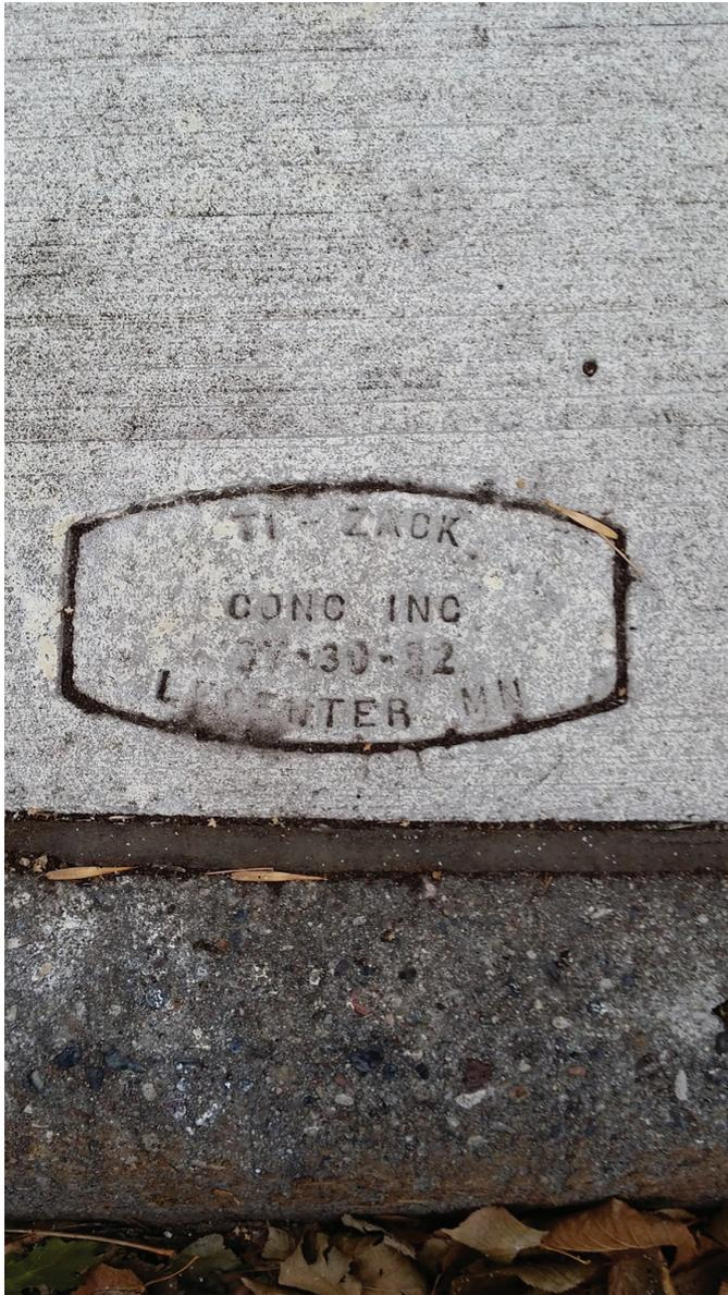
Figure 7. An example of a date stamp on sidewalk replacement/repair. Date is 07-30-12.
