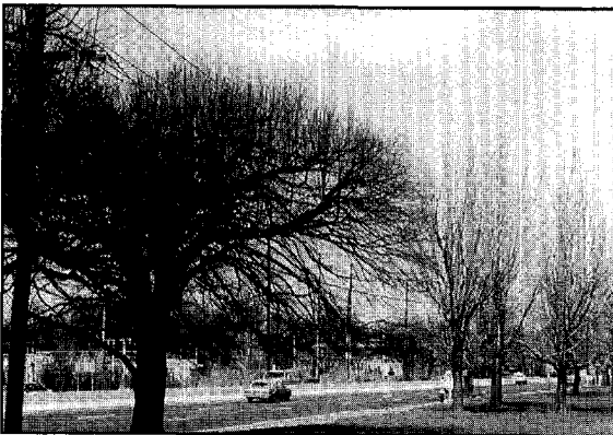
Figure 3. Utility line - street tree conflict solution - off-center planting of fastigiate trees vs. planting directly beneath utility lines. (Right-ginkgo; left-oak)
