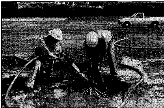
Figure 1. Hydroexcavation of tree roots with a high-pressure water and vacuum system.
