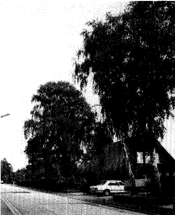
Figure 7. Kungshällagatan is a street built between 1954 and 1956. The sewer line is a combined sewer located in the middle of the street. The problems in this area were caused by trees growing on private property.
