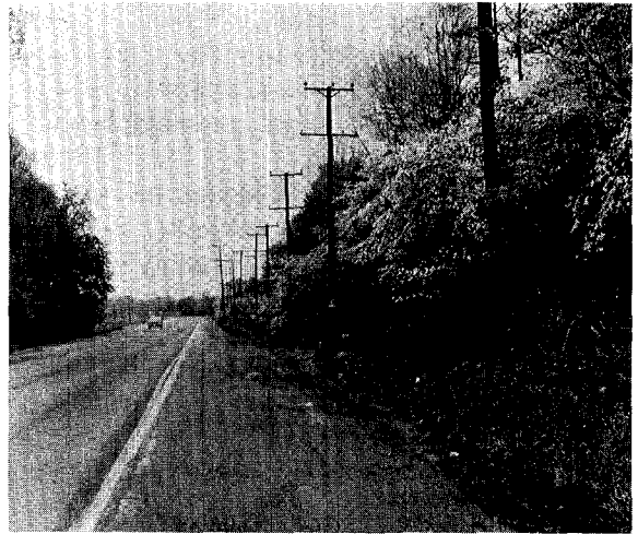
Fig. 5. An aesthetically pleasing community of grasses, herbs, shrubs, and desirable trees under distribution lines.
