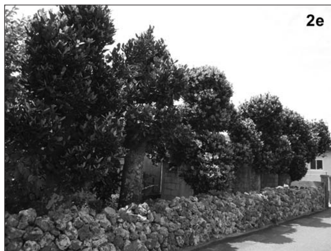
Figure 2e. A huge tree line with the traditional stone fence of coral reef, which were moved inside for the spreading roads. The stone fence was around 1m away from the tree line.
