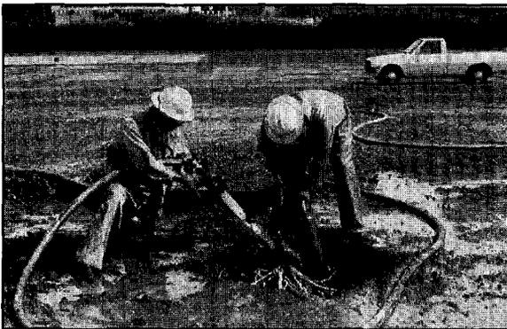
**Figure 1. Hydroexcavation of tree roots with a high-pressure water and vacuum system.**
